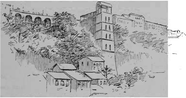
Elevator from the old to the new town, Bahia.
